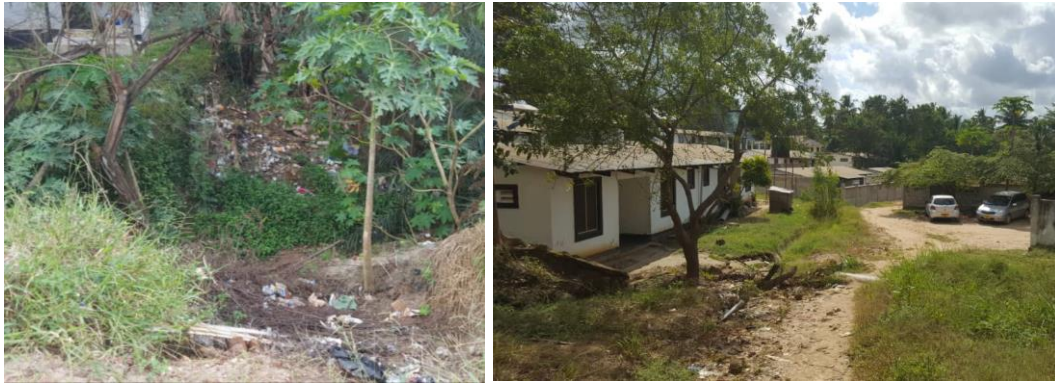
Figure 4: Solid waste dumping area, alleys ( vichocho ), and parking lots at NSSF Housing
